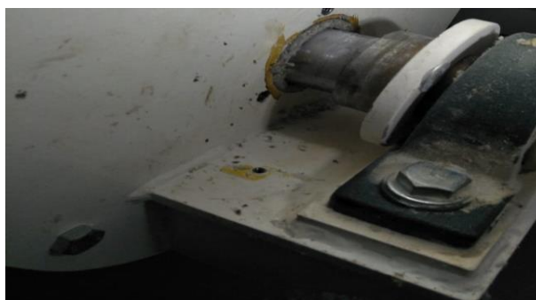
Gambar 9. Pergantian seal gland packing
